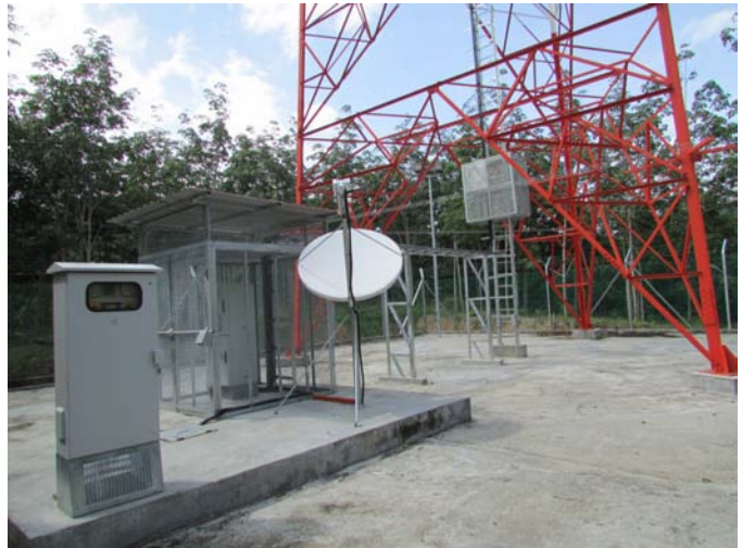
Basic equipment of the Hughes HX system in a cell site in rural Malaysia (photo courtesy of Hughes)
