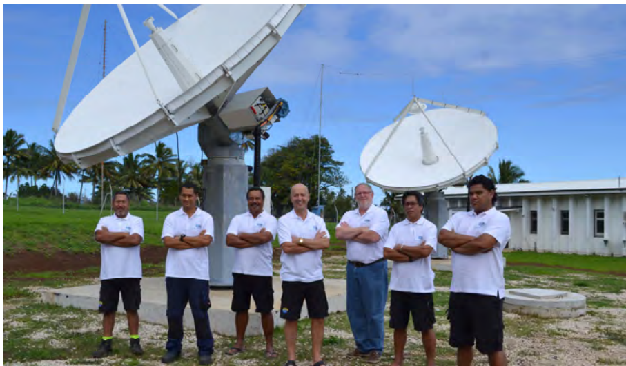
Antennas installed by O3b at the Telecom Cook Islands facility. (photo courtesy of O3b)
