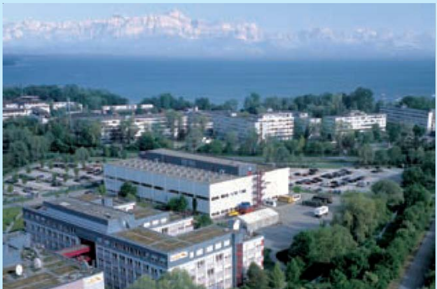
ND SatCom Headquarters in Friedrichshafen, Germany
